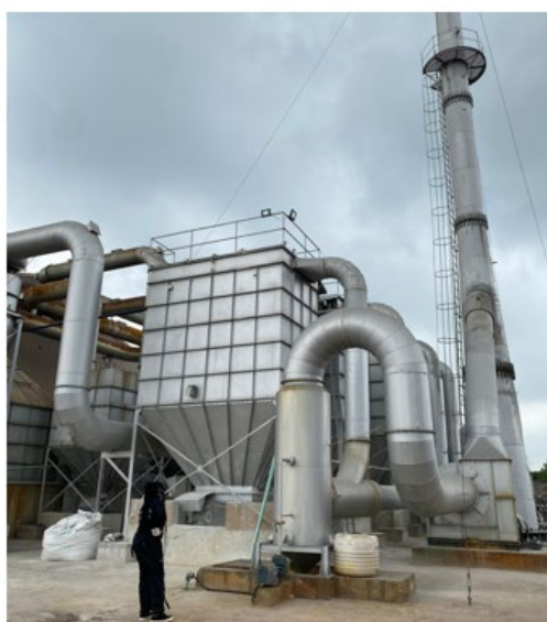
Off-gas treatment system with cooling towers, baghouse, scrubber and stack
